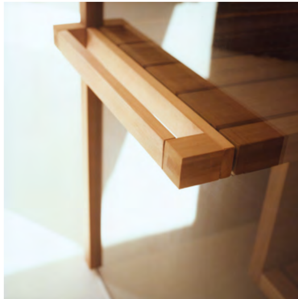
The bench seats project outside, creating a handy towel holder and shelf.
