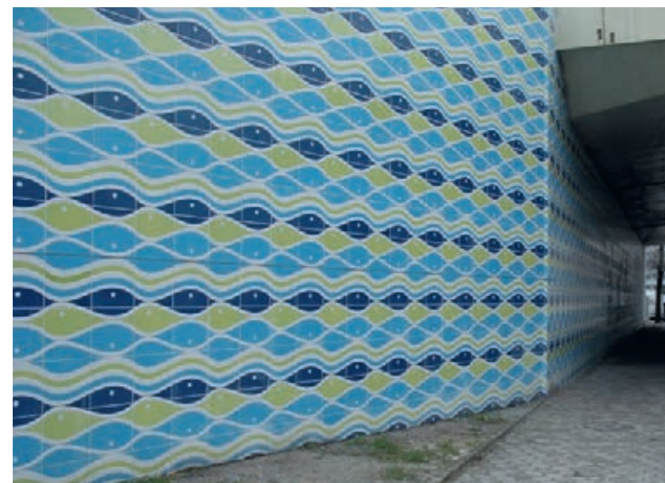
Túnel _ Aveiro, Portugal Tunnel _ Aveiro, Portugal
